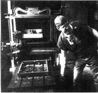
Sanderson operates an 1869 planer. The blacksmith uses mostly machinery that dates to the 1880s and 1920s. He said the state's only other known planer like his is at the Henry Ford Museum in Dearborn.
